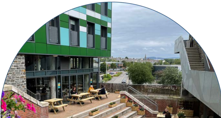
Coastal's 'Urban Village' regeneration scheme on Swansea's High Street brings together social housing and a mix of commercial premises let to independent retailers, creative industry and tech companies.
