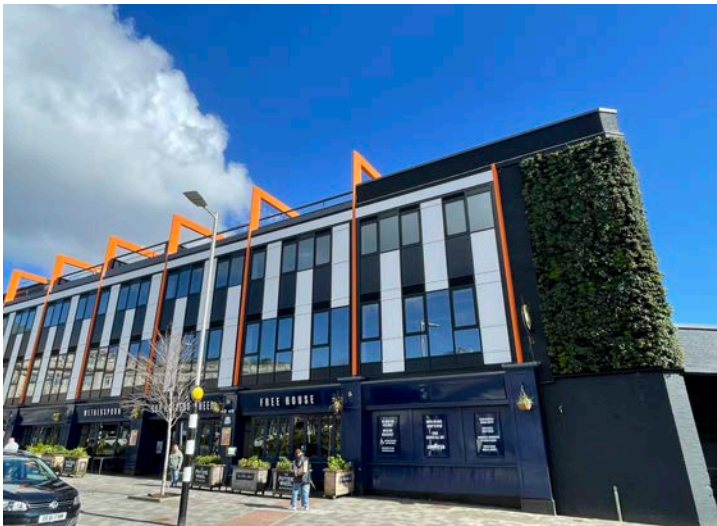
Our upgrade of 85 The Kingsway in Swansea features the city centre's first living, green walls.
